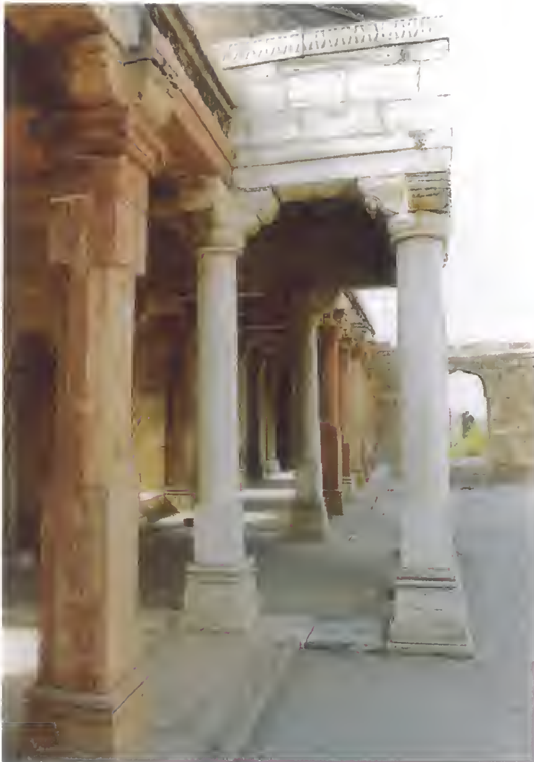
The roof of Sultan Ghari's tomb at Delhi which was once a temple, then a mosque and now both
